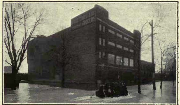
George C. Buell Company's Warehouse, Rochester, N. Y. Walker, Livingston & Brackett, Architects
